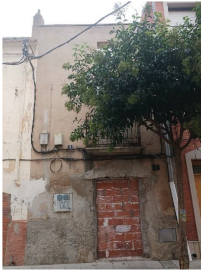
f5_façana principal Miralles, 9
