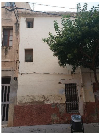
f3_façana principal Miralles, 7
